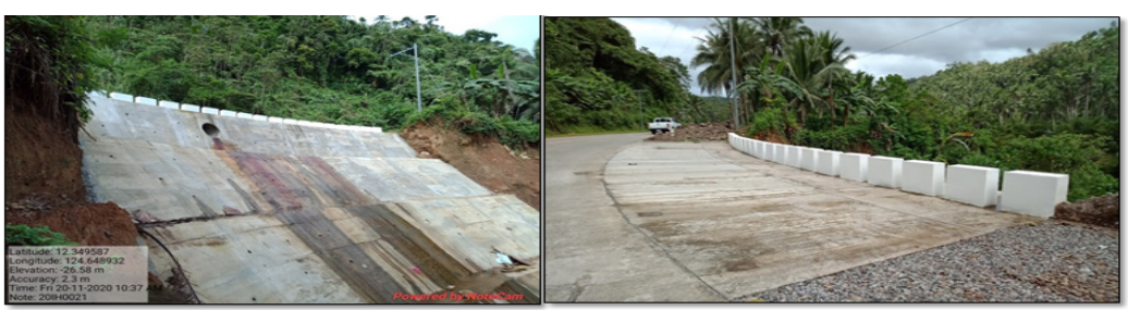
Brgy. Cervantes Slope Protection K0765+460-K0765+480)
