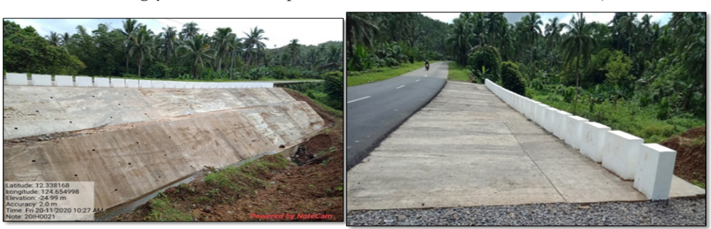
Geratigan Slope Protection (K0767+473-K0767+505)
