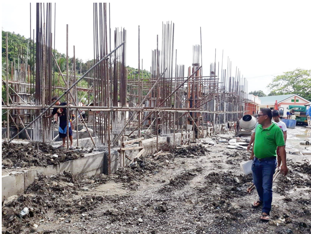
Wilfredo Mosong, school head of Liloan National Technical Vocational High School, supervised the ongoing construction of project. Ongoing activity in the project site include pouring of concrete for the tie beam.
