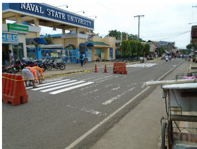
Repainting of pedestrian lane in front of Biliran Province State University (BiPSU) main campus, former Naval State University (NSU) to provide a safety lane for students when crossing the street.
